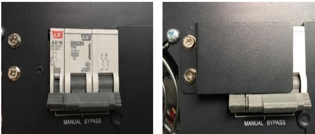
Figure 6 Breaker and baffle installation
