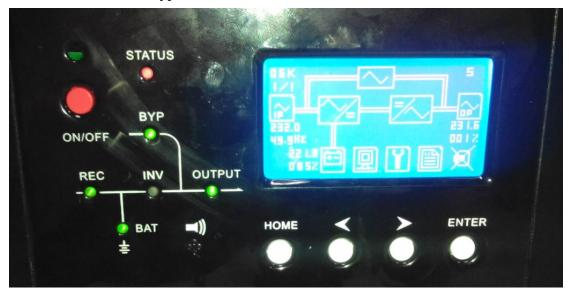
(1) Remove Maintenance bypass circuit breaker cover3 in condition of normal mode, UPS transfer to bypass, then close Maintenance bypass breaker. And the load is powered through maintenance bypass and static bypass.
