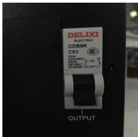
Figure 5 Breakers and baffle installation
