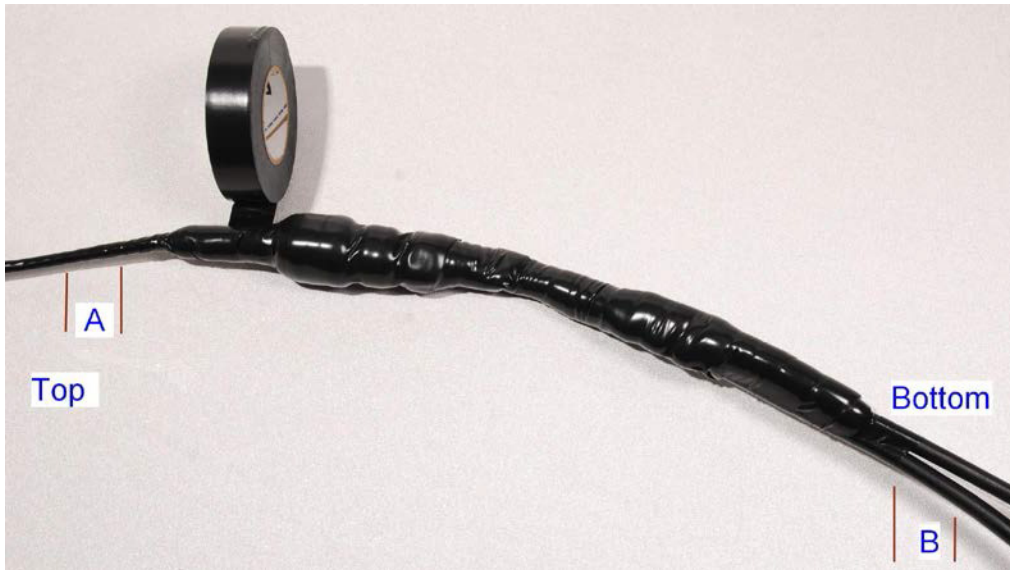
Figure 107 Wrapping PVC tape around the GPS adapter cable joint
