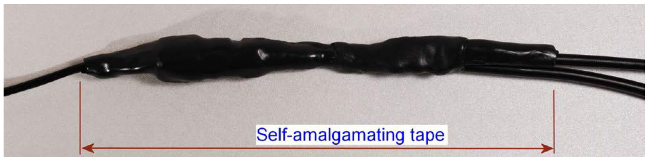
Figure 106 Wrapping self-amalgamating tape around the GPS adapter cable joint
